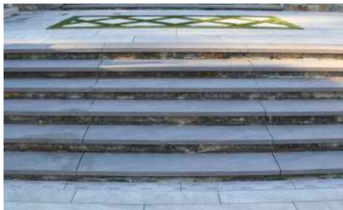
Mitered steps and custom drains
